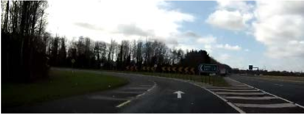
Photo 7 N6 Dual Carriageway Westbound Exit at Junction 12 (from Dublin)
