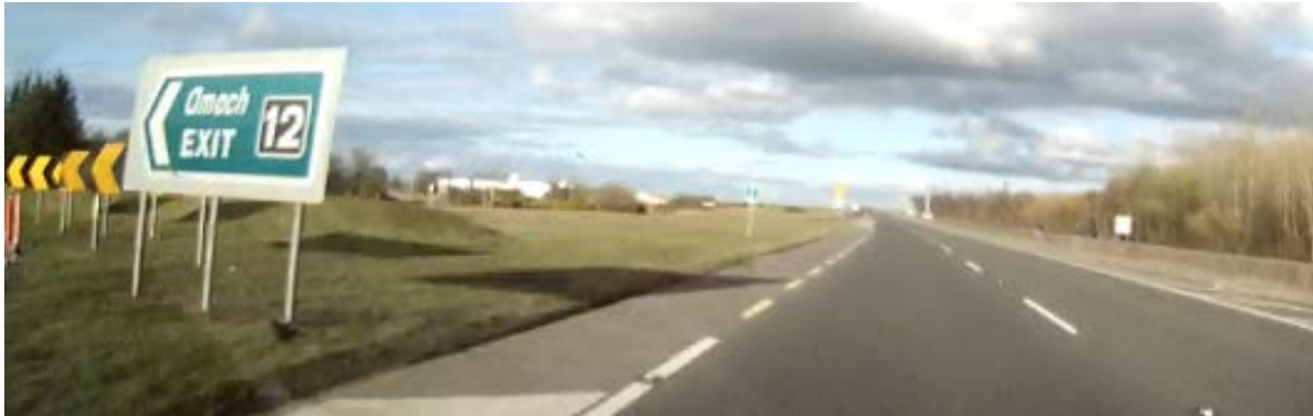
Photo 2 N6 Dual Carriageway Eastbound east of Junction 12 Exit
