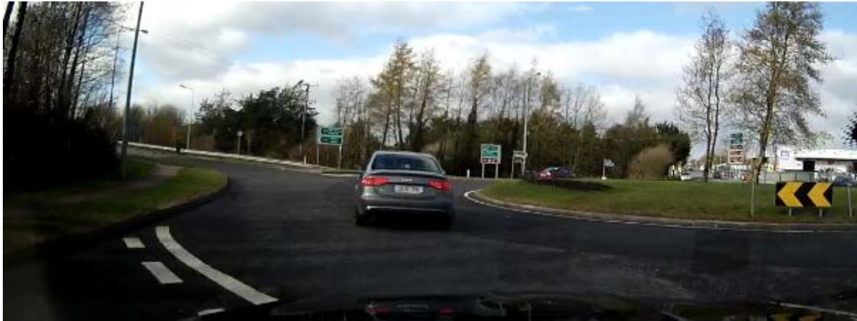
Photo 3 Ganly's Roundabout N61 Northbound view at the exit onto the Roundabout
