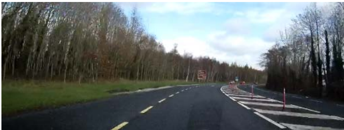
Photo 9 N6 Slip Lane between Junction 12 Exit and T-Junction with N61 / R914
