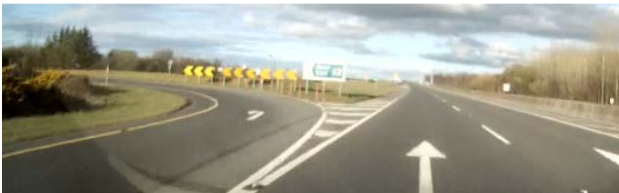
Photo 1 N6 Dual Carriageway Eastbound at Junction 12 Exit (from Galway)
